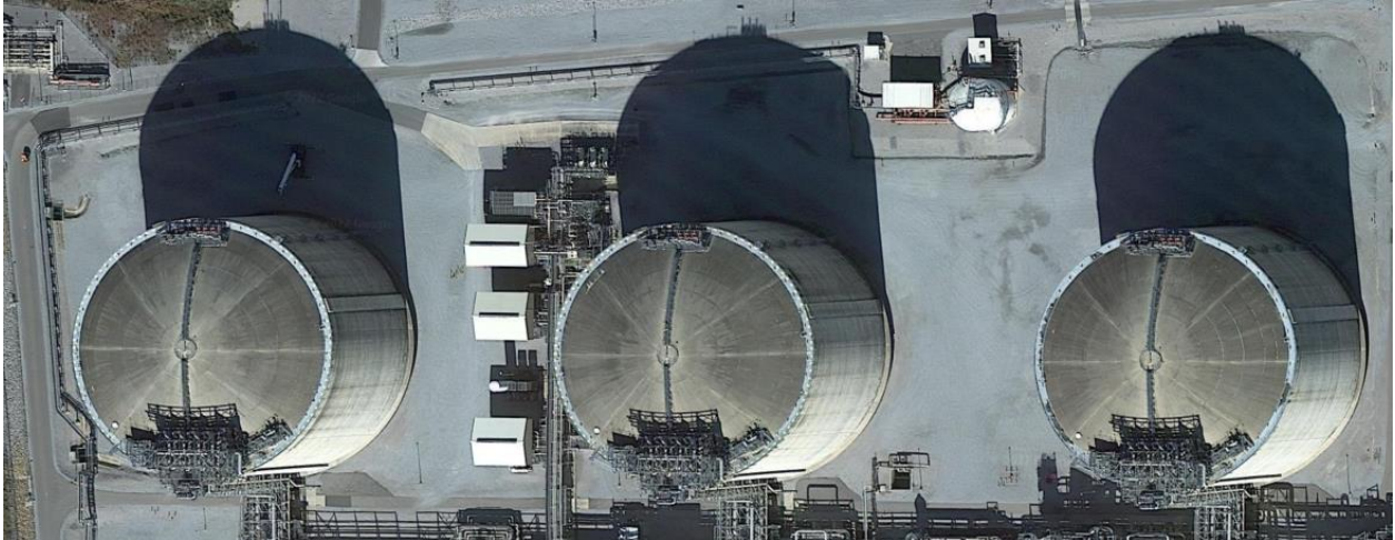
Figure 19: Three full containment LNG tanks
